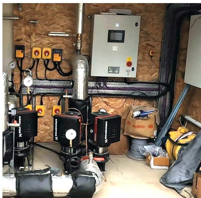
Efficiency is further enhanced through the tracking of five buffer sensors and multiple pipework points, to avoid short cycling and give smooth, efficient performance with full visibility in the cloud.
