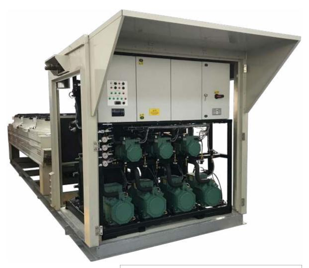
Duty range is 70-320kW and is offered as a dual temperature solution.
